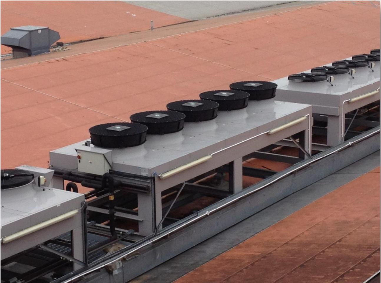
An AxiTop trial was conducted by Space Engineering Services and Coolers and Condensers on behalf of a major UK supermarket with the aim to evaluate what energy saving benefit was available by retrofitting existing EC condenser fans with the new AxiTop diffuser.
