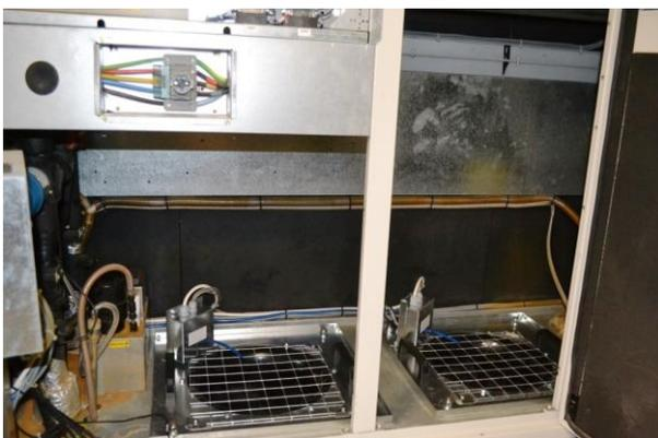
Two off EC backward curved fans, positioned in the floor void.
