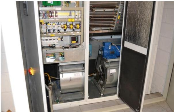
Two off AC forward curved belt drive blowers, positioned inside the unit.
